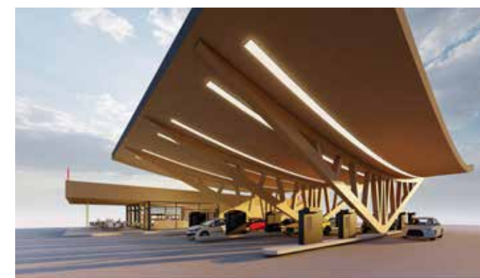
Trusses made from glulam help to create a great room at an ordinary gas station canopy.
