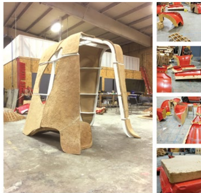
The final cast wood pavilion is shown here with the vinyl taped forms into which the wood mixture was cast.
