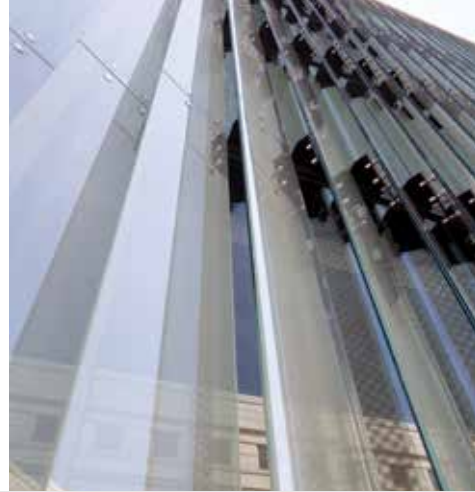
Left: A series of frosted glass fins covers the western facade of the addition. Middle: The arched windows of Vol Walker Hall were restored during the project. Right: A craftsman touches up the molded plaster in the second floor gallery. Opposite page: Left: Glass-walled fire stairs connect Vol Walker Hall and the Anderson Design Center addition. Right: This plan details the landscape strategy for the project.
