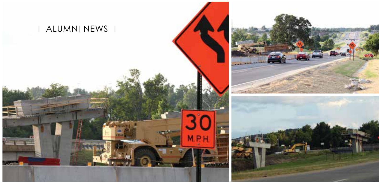
The flyover bridge in north Fayetteville will provide direct access from College Avenue to I-540, so northbound drivers don't have to make a U-turn at the Joyce Boulevard traffic light. Construction could continue until early 2015.
