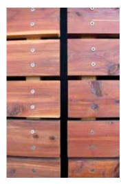
A mark of precision, screw heads are positioned the same way on the cedar screen.
