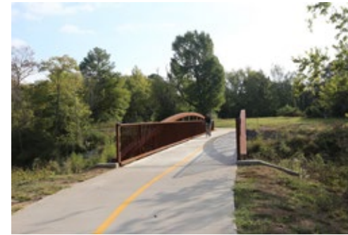
Long bridge on the Cato Springs Trail
