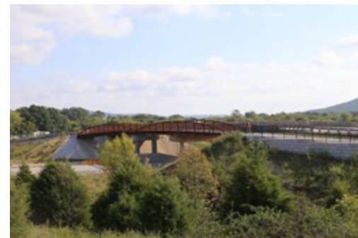
Bridge over the Fulbright Expressway, Cato Springs Trail. Photos by Dede Peters
