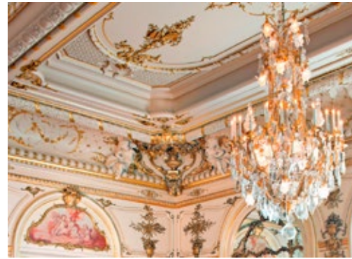
Restoration finishes are completed
